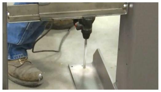
**6.** Pound in the 10 Red Head Anchors. The length of the anchors depends on the thickness of the concrete.
