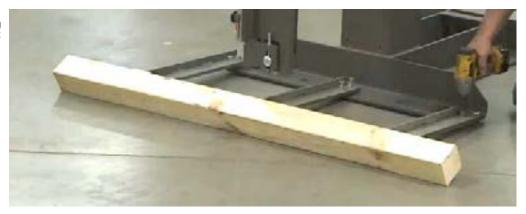
**5.** Using a hammer drill, drill the mounting holes in the floor with the correct drill bit to match the mounting hardware.
